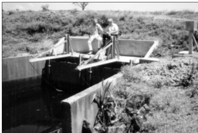
Caption2: Wants Drain After Installation of Lifting Winches
