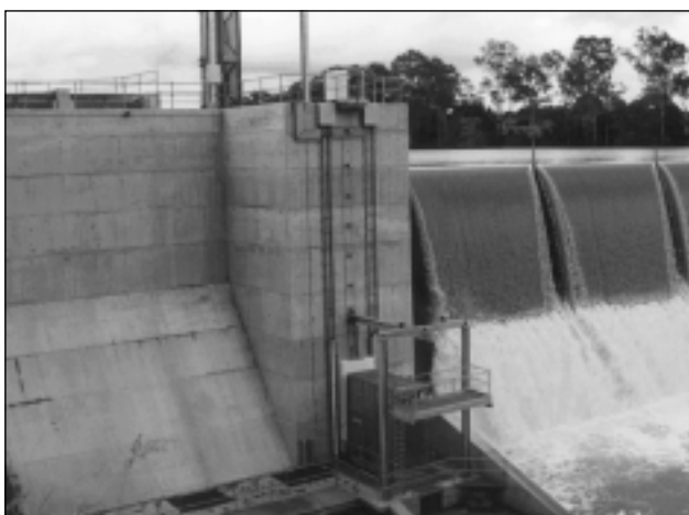
Figure 8: Fish Lock at Walla Weir near Bundaberg
