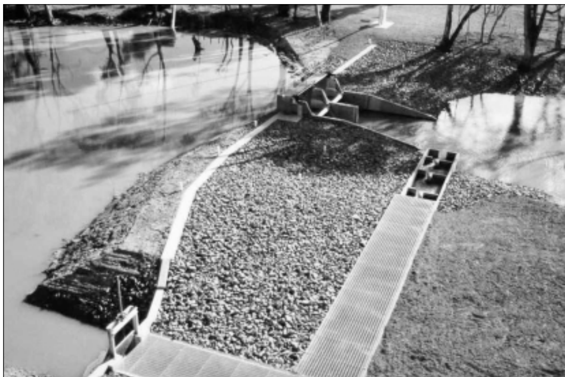
Plate 4: Typical New Weir and Fishway
