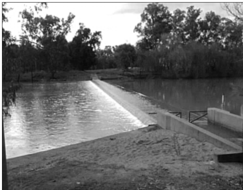
Figure 2b: Weir types in the Murrumbidgee. Overshot weir. Yanco Weir.
